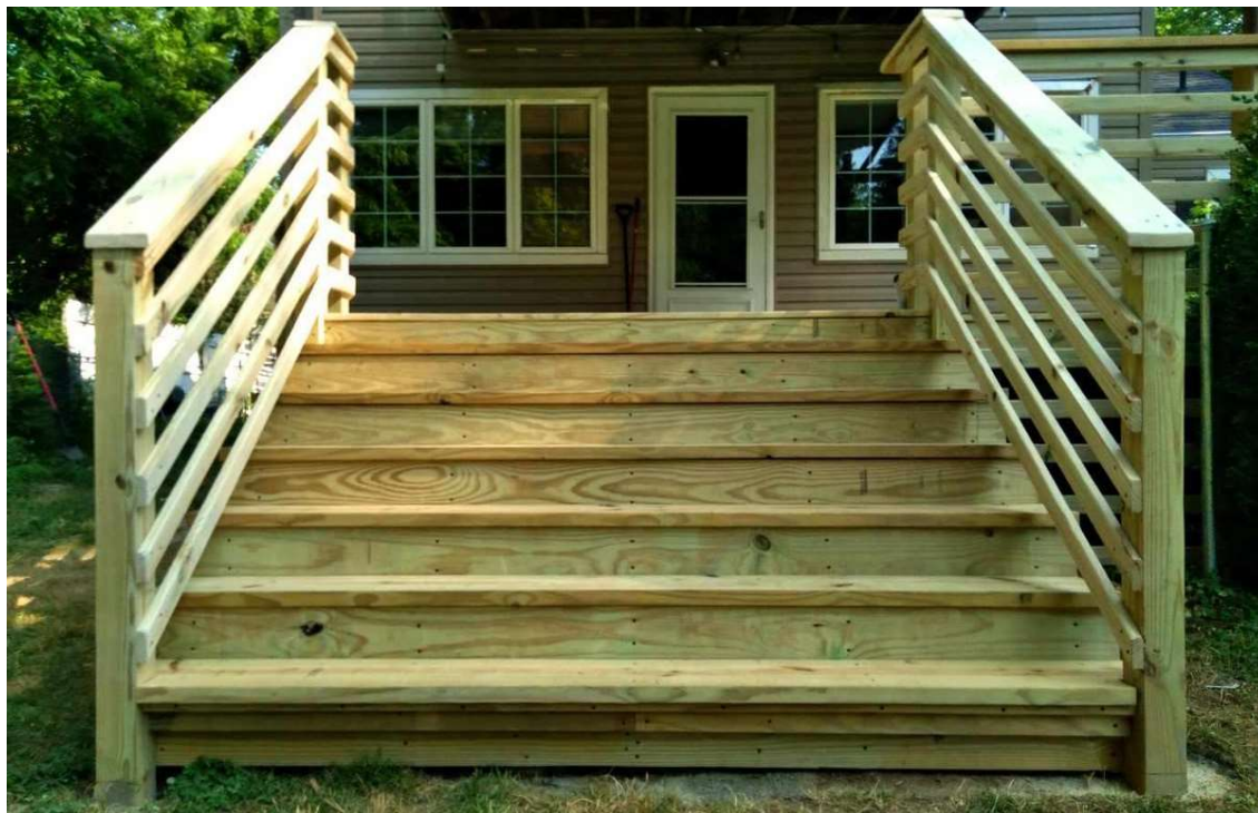
Pictures from the Dumas deck project
