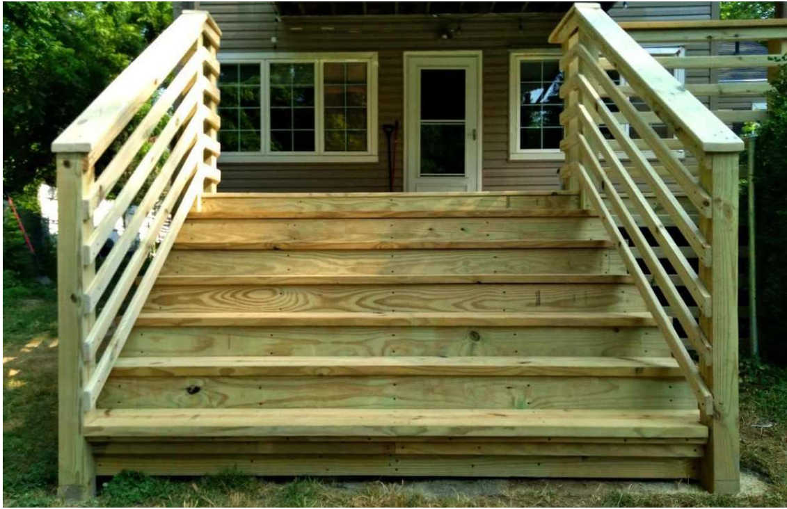
Pictures from the Dumas deck project
